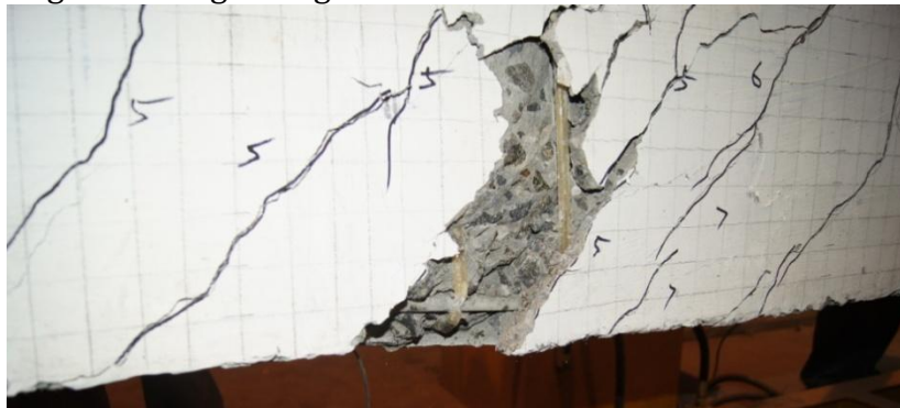
Figure 8: Failure of GFRP reinforced rectangular beam due to excessive spalling of cover followed by concrete crushing ( Bp_1m_1F_t )
